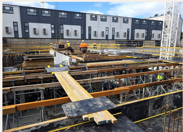
FORMWORK · MOORABBIN · 2025 Cardabuilt — Moorabbin
