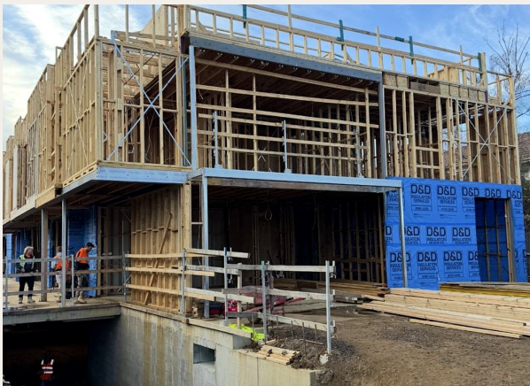
MULTI-RESIDENTIAL · BRIGHTON · 2025 D5 Build — Brighton
